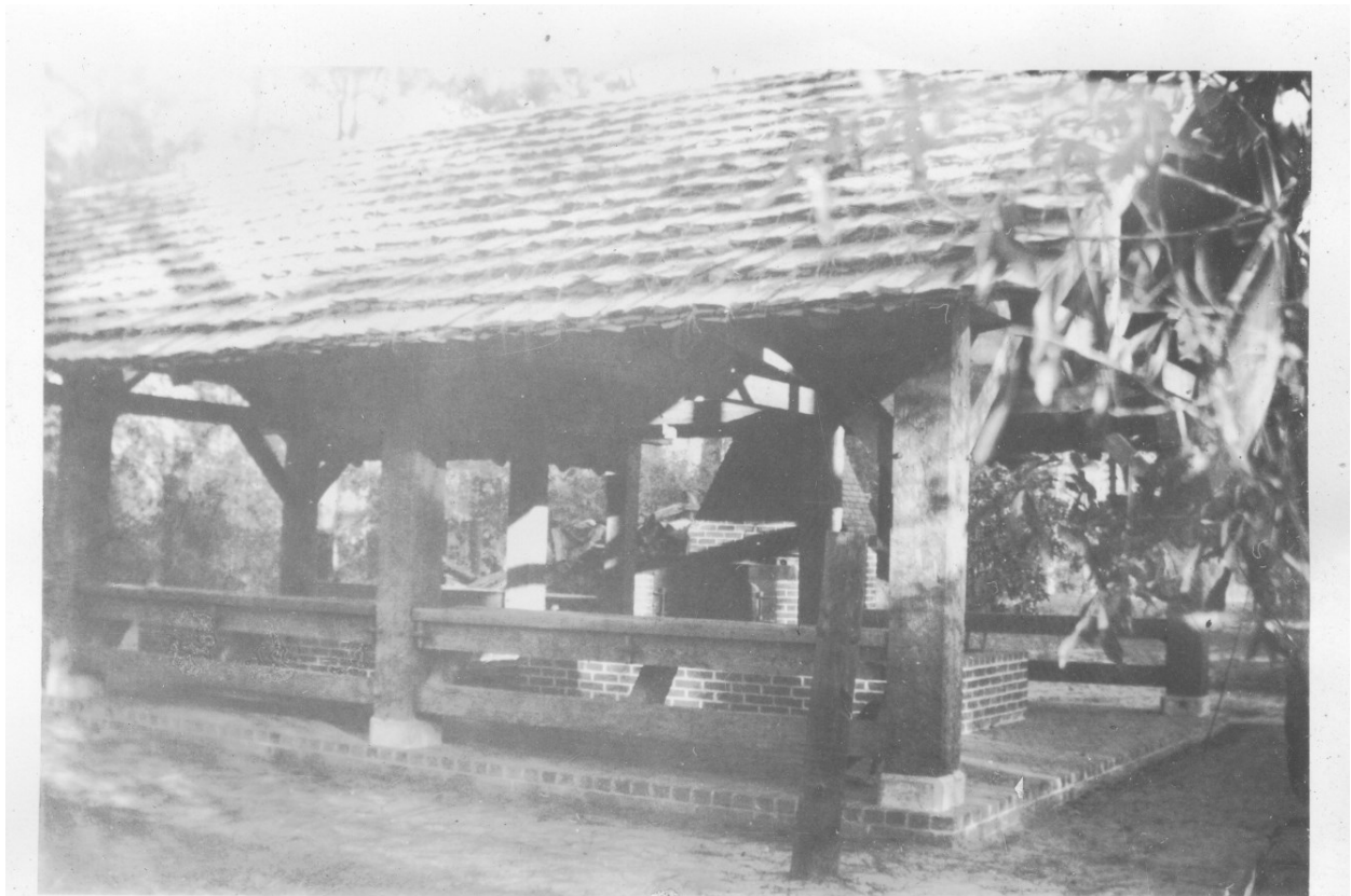
This shelter was built using timber from the park. The enrollees also made the cypress shingles. (photo courtesy of B.R. Caldwell)
